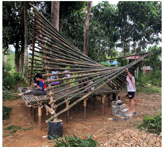
Picture shows before and after of the pavilion construction process.
